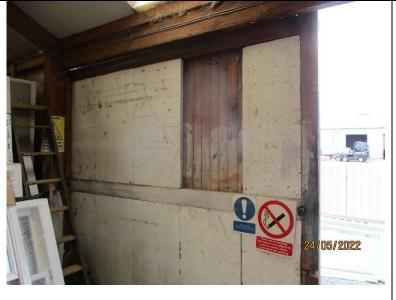
This is despite poor insulation and sound insulation, and with a panel missing from the door.
